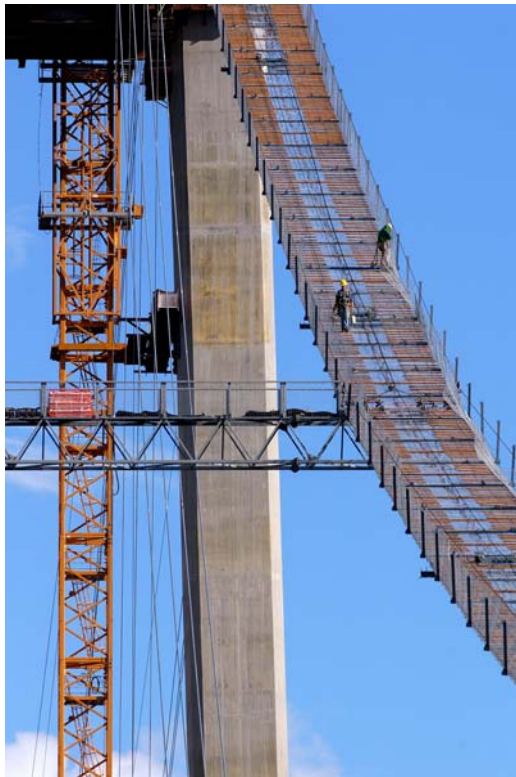
Tacoma Narrows Bridge Location: Tacoma, WA Photo Date: 8/1/2005
