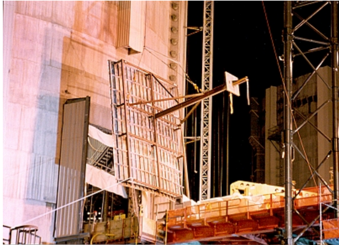
Nuclear Steam Generator Replacement Location: Byron, IL Photo Date: 1996
